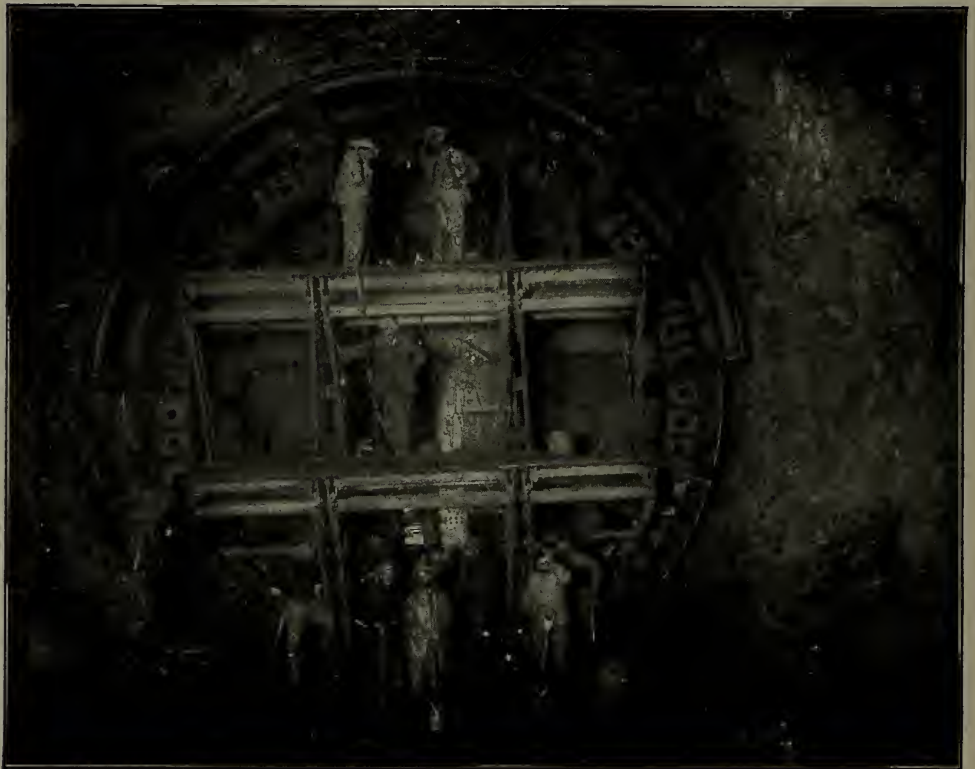
Shield Fitted with Fixed Hoods and Fixed Extensions to the Floors.
